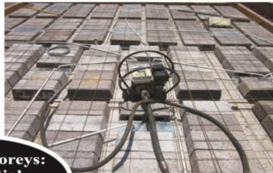
Lattice Beam Slabs
